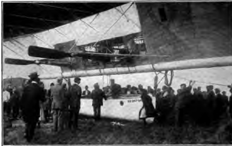
Fig. 24. View of Car Showing Propellers and Canvas Covering
